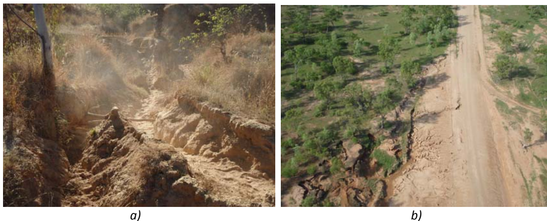
Figure 10 Examples of a) a cattle pad cut down a steep river bank that is rapidly being transformed into an alluvial gully, and b) an alluvial gully initiated by a poorly designed road crossing a river.
