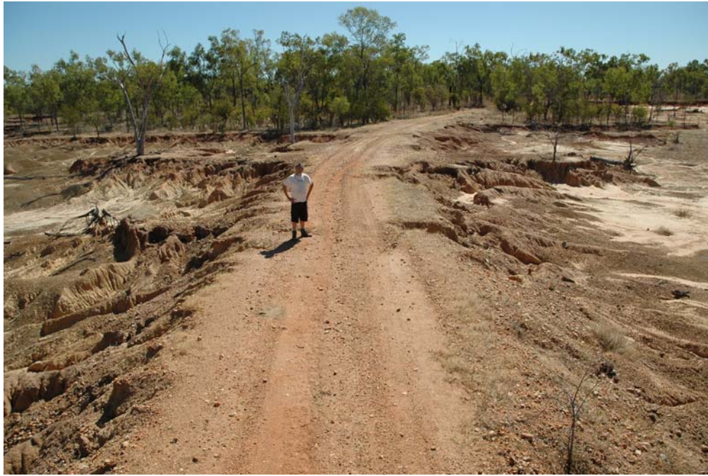
Figure 4 A road located on the apex of an floodplain alluvial ridge that has been consumed by the merging of proximal and distal draining gullies. Note that in this situation, just direct rainfall and local runoff are needed for headward retreat that progresses until none of the original floodplain surface remains.
