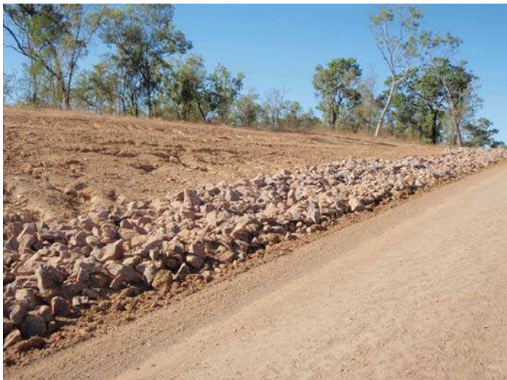
Figure 7-3 Road slope bank after two wet seasons in 2009. The gully in the road ditch was armoured with rip-rap, and rilling on the largely unvegetated cut bank continues.
