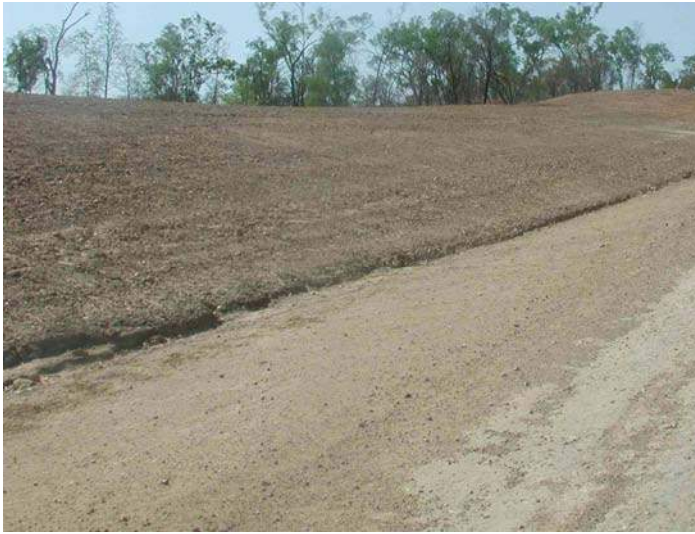
Figure 7-1 Road cut slope after initial re-grading in 2007 and one initial rainfall event.
