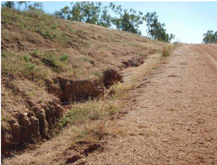
Figure 7-2 Road cut slope after one wet season in 2008. Note rilling and gullying.
