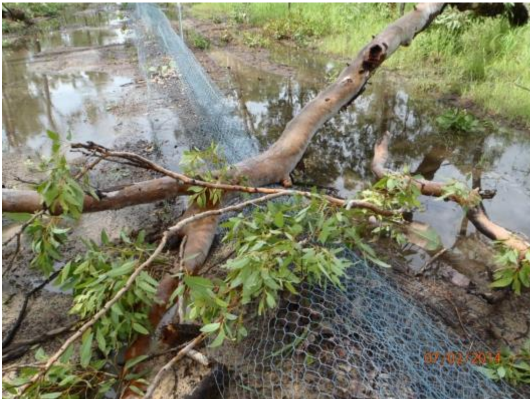
Figure 5. Fence damage caused by a fallen tree (photo Khan Spokes)
