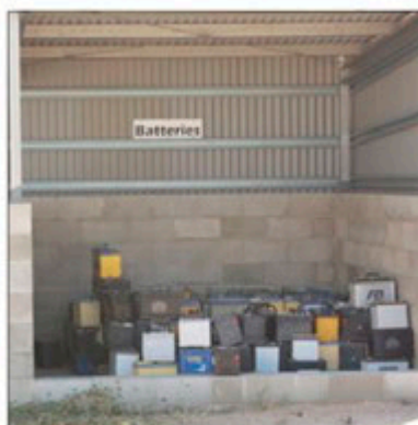
Batteries stored in bunded shed Pormpuraaw Aboriginal Shire Council, Sept. 2016
