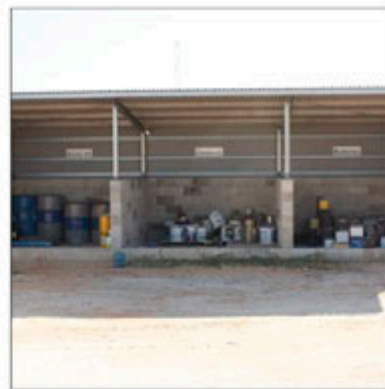
Pormpuraaw landfill site - banded undercover storage for hazardous waste, Sept. 2016
